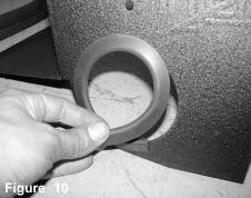
Install the vinyl trim to the hole cut out on heat shield.
